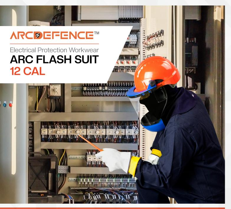
Arc Defence™ by Hicare light weight Arc Flash Protection, an arc flash occurs when the electrical current flows outside its intended path, through an air gap, to another conductor. With this in mind, you can see that an arc flash can occur anywhere that the electrical current has a chance to escape. Arc flash suits are full-body protective garments required for electrical workers to protect them from the heat and energy released during an arc flash.
